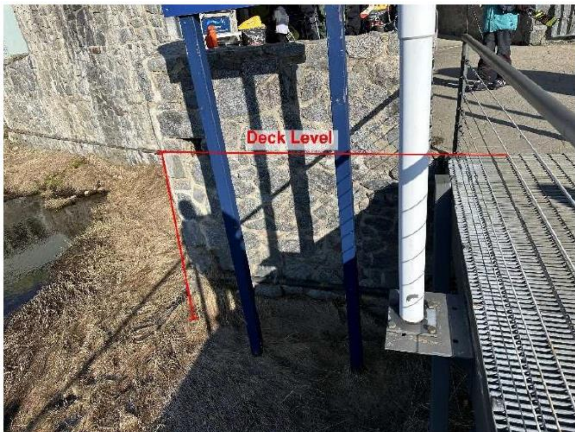
Figure 5 | Location of works in relation to Perisher Creek (Source: Applicant's documentation)
