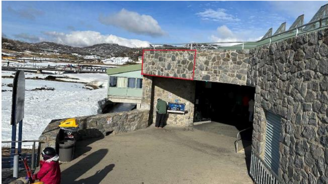
Figure 4 | Lower-level entry location for proposed lift, showing approximate section of existing rock wall to be removed (in red) allowing for exit/entry of the lift at the upper deck level (Source: Applicant's documentation)
